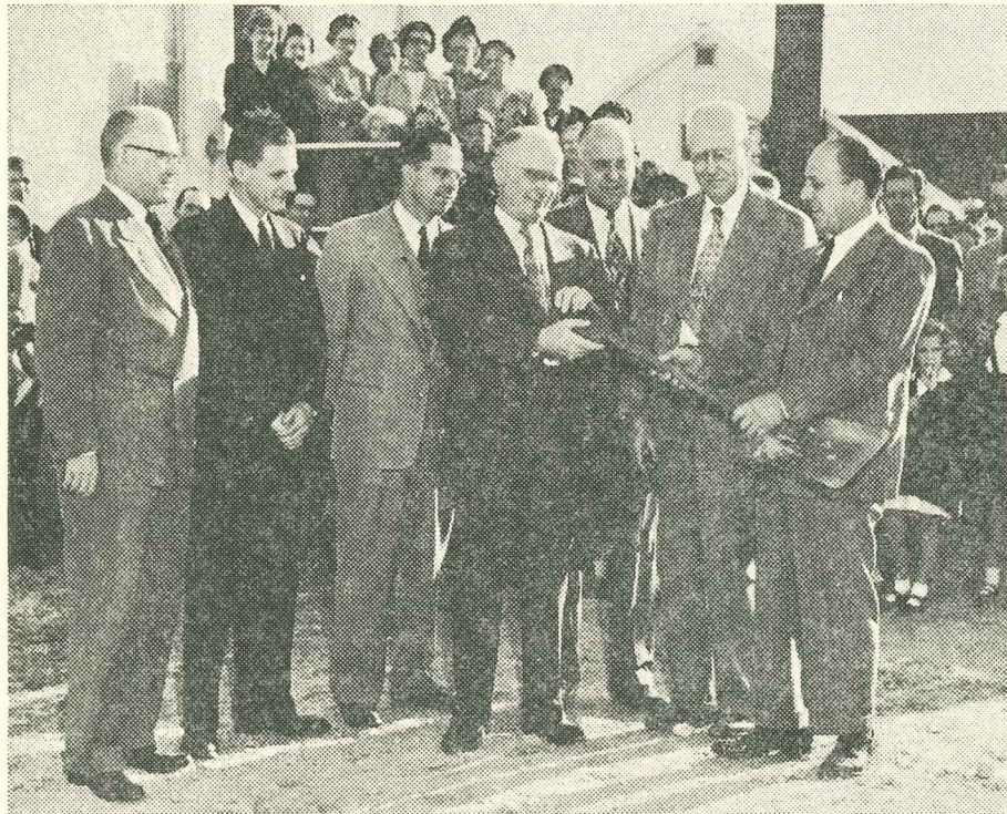
Dr. O. W. Yates, pastor of the Rosemont Baptist Church of Lexington, is shown getting a shovel from Frank Happ, associate chairman of the church's building committee, Sunday afternoon as he prepared to move the first shovelful of dirt for the foundation for a new church building. Work on the foundation is expected to start in a few days. Construction of the building proper is scheduled to get under way next spring. Principal speaker for the occasion was Dr. F. Russell Purdy, shown at left, pastor of the Calvary Baptist church, Lexington. Others, left to right, are William Mitchell, Rosemont music and educational director; the Rev. Ira McMillan, pastor of Hillcrest Baptist Church; Mr. Yates; the Rev. O'Ray Weeks, pastor of Porter Memorial Baptist Church; Charles Hatfield, clerk of the Elkhorn Baptist Association, and Mr. Happ.—The Lexington Leader.
