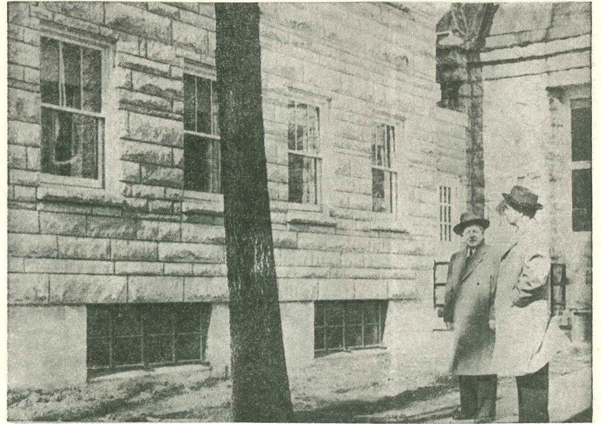
J. Smith Barlow, chairman of the Building Committee, and Pastor C. Carman Sharp standing in front of the new Bardstown Baptist Educational Building looking it over. It is made of white limestone.
