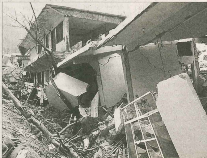
HOUSING NEEDED Southern Baptist volunteers are helping build temporary shelters to provide relief from the harsh winter.
