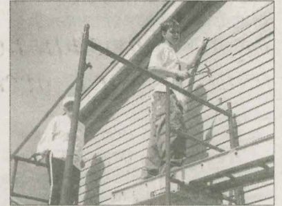
SIDING Josh Price (right) secures vinyl siding. He is the son of Valerie Price, the new homeowner. The project was done in cooperation with Habitat for Humanity.
