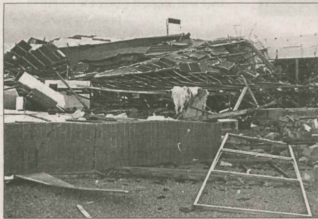
Total loss North Livingston Baptist Church, in Hampton, was destroyed by a tornado Jan. 12. (Photo provided by Danny Starrick)
