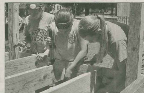
Volunteers begin assembling a deck for a homeowner in Campbellsville. From left are Carley Johnson, Jaley Broughton and Peyton Ingram, all from Eubank Baptist Church in Eubank. (Photo by Lauren Barr)
