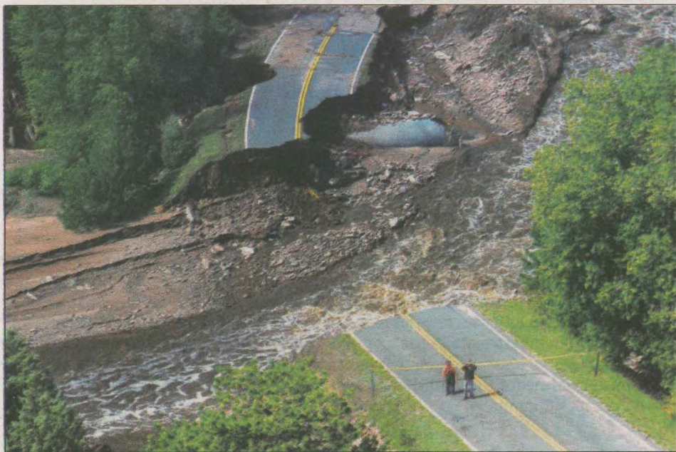
An aerial view shows the extensive damage to a road in Colorado due to flooding in mid-September. (Photo/U.S. Army Sgt. Jonathan Thibault)
