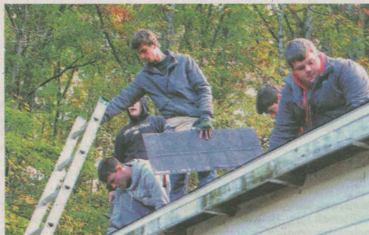
Campbellsville University Repair Affair students work on a roof with Kentucky Heartland Outreach.
