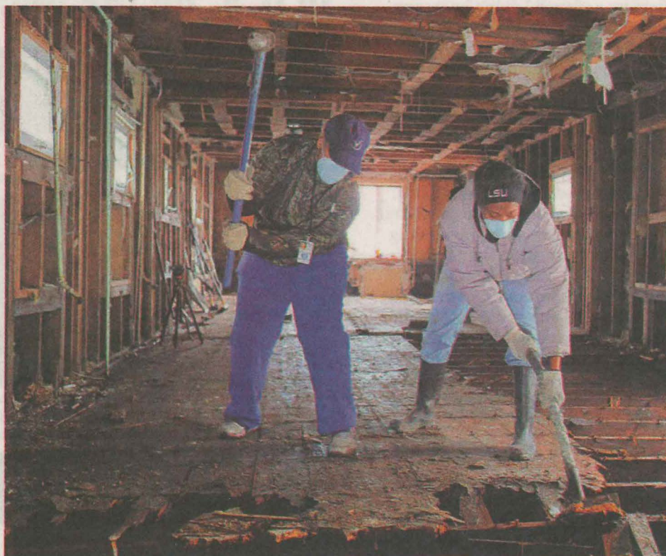
Louisiana State University students Skyler Hollins (left) and Taylor Christian wield sledgehammers to remove flooring from a Staten Island home flooded by Hurricane Sandy's storm surge. More than 500 students volunteered part of their winter breaks to work with SBDR volunteers last year. Registration for this year's Sandy Rebuild effort is now open for spring breaks and summer. (NAMB)
