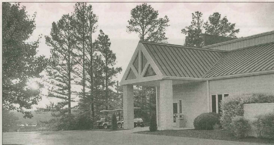
Jonathan Creek's new worship center built this year still has a few finishing touches that need completing, but summer counselors for Crossings at the Creek still met for the building's dedication. More than 12,000 students will pass through and worship in the building this summer. (Photo by Whitney Jones)
