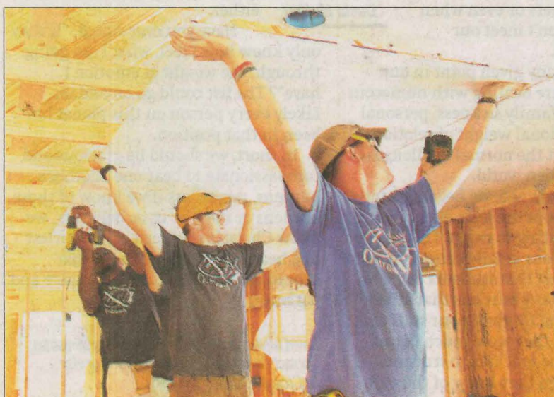
University of the Cumberlands football players Iquan Deed (left) and Chad Bond (center) join former Patriot Justin Dyer in hanging drywall at one of two homes that the university's Mountain Outreach program are building this summer. (UC photo)
