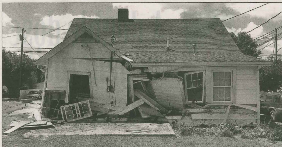
The now-condemned Waddy Baptist Church parsonage awaits demolition after a 75-foot water tower struck it when it fell Aug. 9. The 100,000 gallons of water in the tower also flooded the church's basement and the nearby post office. (Photo by Todd Deaton)
