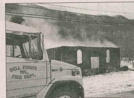
Fire destroyed the sanctuary of Mill Creek Baptist Church on Feb. 18. Only the basement walls and outer walls of the sanctuary remain.
