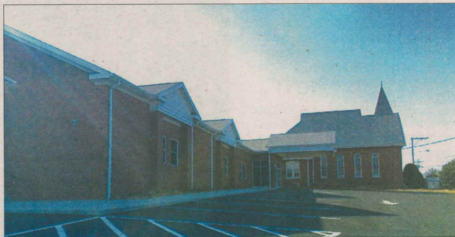
Corydon Baptist recently completed a $1.2 million education and fellowship facility.
