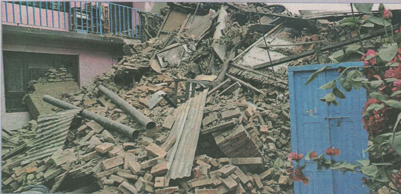
Many buildings around Kathmandu are reduced to rubble in the aftermath of the 7.8-magnitude earthquake April 25. (Photo used with permission)
