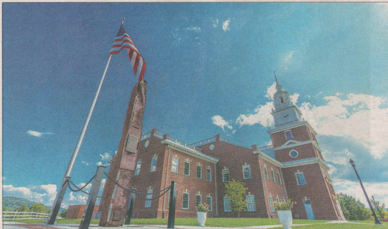
A beam from Ground Zero in New York City stands tall on the campus of University of the Cumberlands in Williamsburg.
