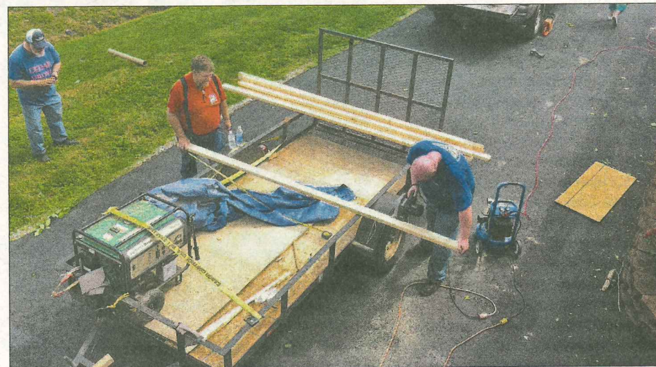
Disaster relief crew members improvise with a trailer to cut boards for repairing the roof of Cedar Grove Baptist Church.
