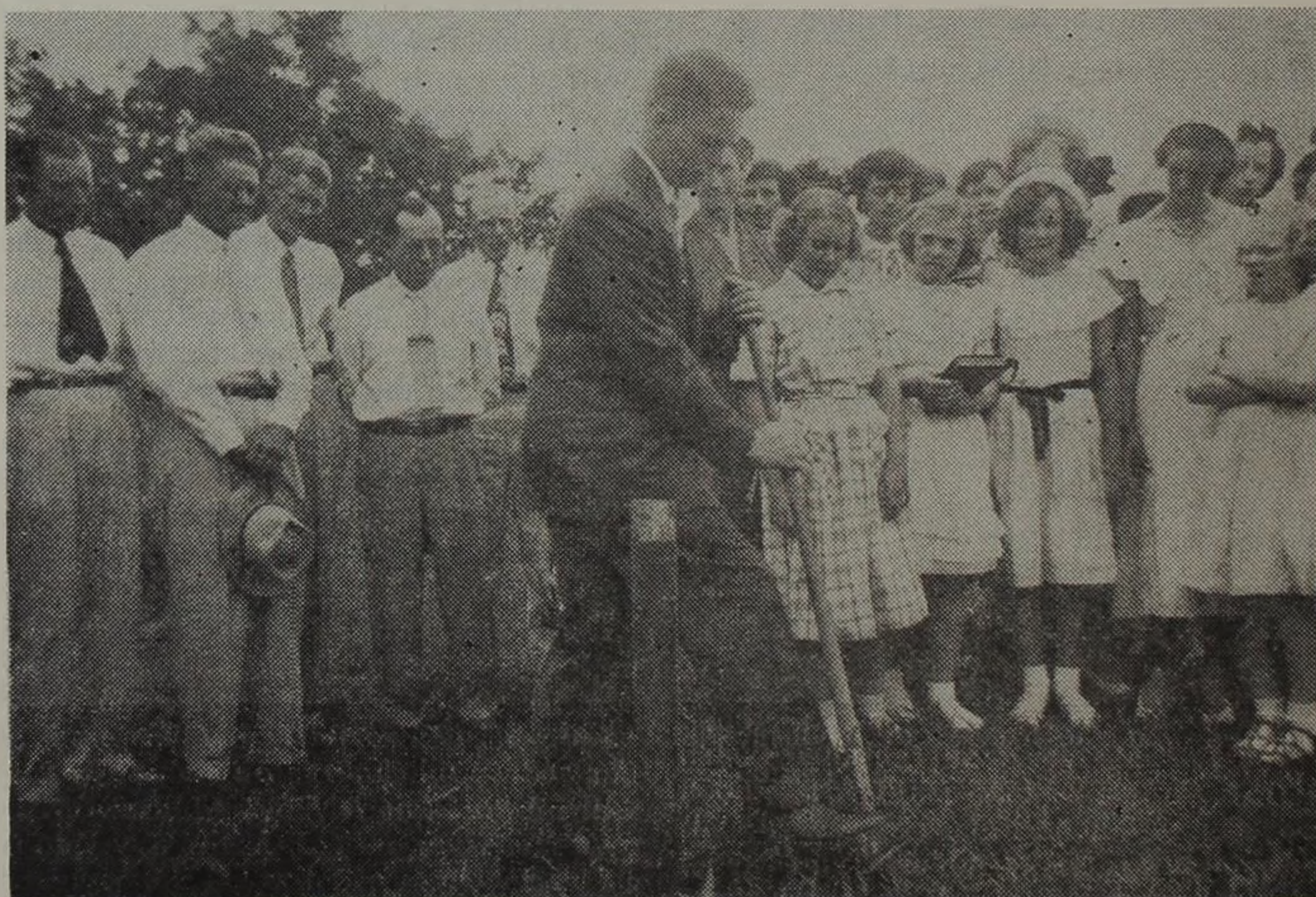
Pastor Jerold Palmer, Jr., is shown breaking ground for the pastor's new home of Bethel church, near Humboldt. Others on the building committee are Herndon McLeary, J. W. Todd, Alex Kyles and Howard Blurton.
