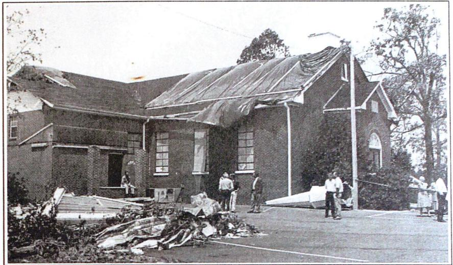
**MEMBERS OF Park Grove Church, Ethridge, assess the damage done by tornadoes last week in Lawrence County. In addition to the steeple on the ground, the roof was badly damaged and bricks were torn off the rear wall of the church. Trees also were uprooted on the church property.**
