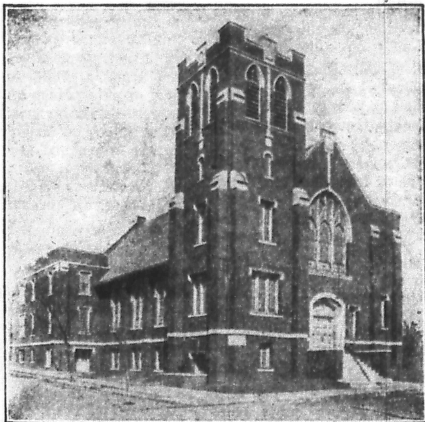
HIGHLAND PARK BAPTIST CHURCH
