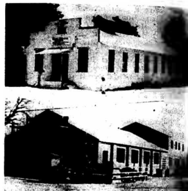
(upper) Church building from 1947-1950 (lower) New building under construction (above right) New home Antioch Church
